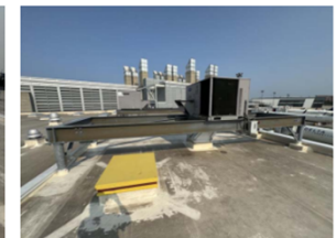
PHOTO 6: STEEL DUNNAGE ON ROOF AREA E.
