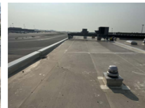
PHOTO 5: PARTIAL VIEW OF ROOF AREA E.
