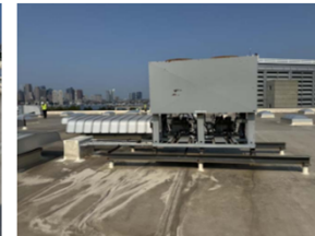
PHOTO 2: STEEL DUNNAGE ON ROOF AREA A.
