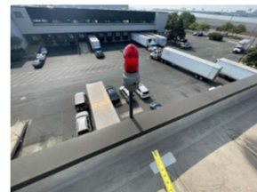
PHOTO 4: TYPICAL PARAPET ON ROOF AREA A.
