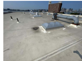
PHOTO 1: PARTIAL VIEW OF ROOF AREA A.
