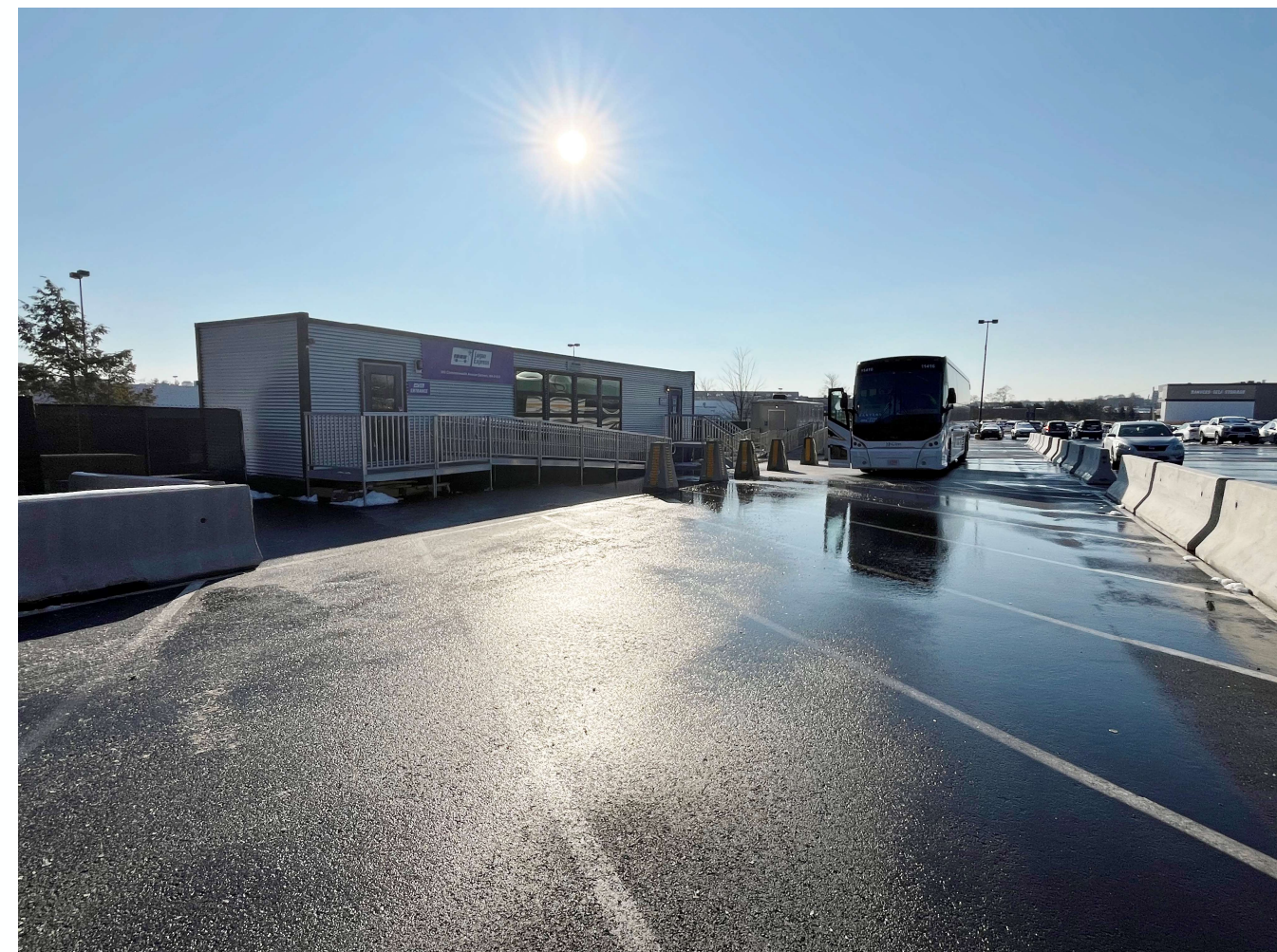
VIEW OF TICKETING OFFICE TRAILER AND BUS LANE
