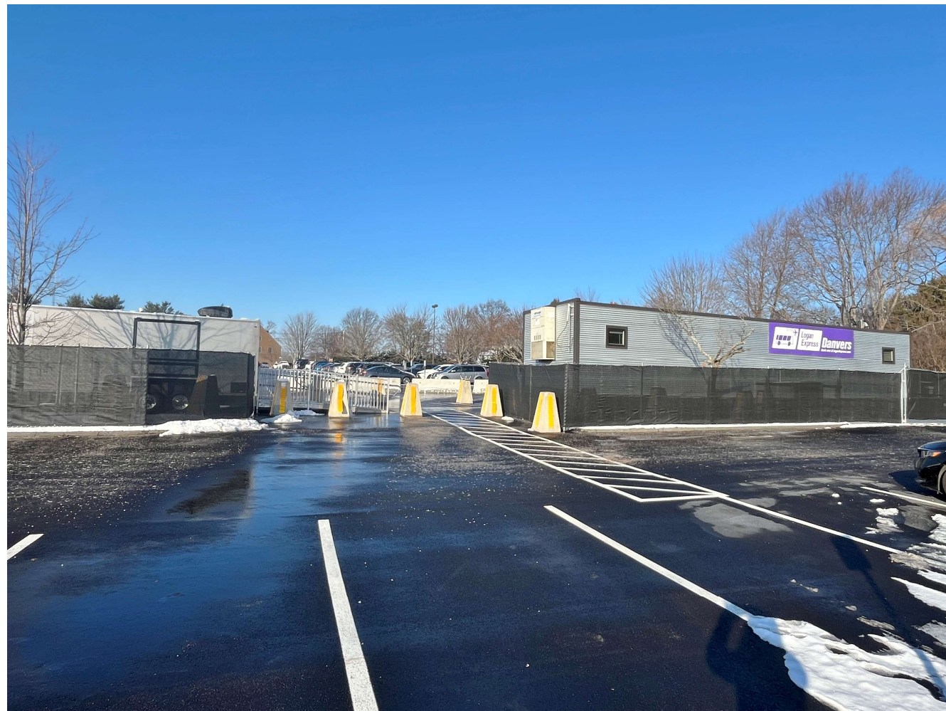
VIEW OF PEDESTRIAN WALK AT SHORT-TERM PARKING LOT
