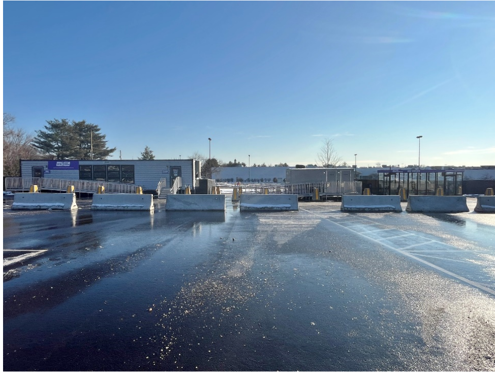
VIEW OF TICKETING OFFICE TRAILER, RESTROOM TRAILER AND BUS SHELTER
