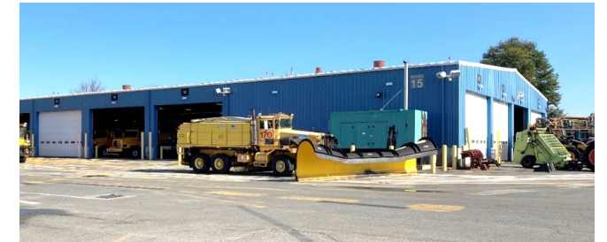
Building 15 – Large Vehicle Storage
