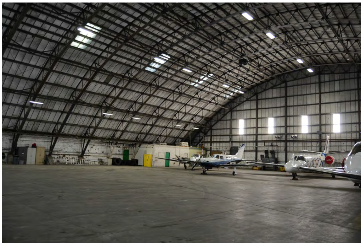
Photo 3. Interior, view looking east.
