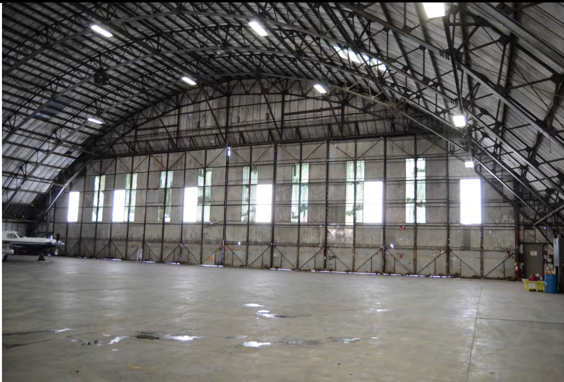
Photo 4. Interior, view looking west.
