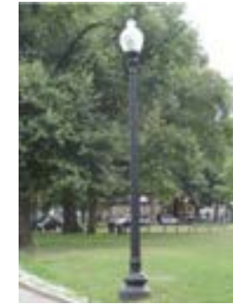
Acorn Style Pedestrian Pole Light approximately 15 feet high
