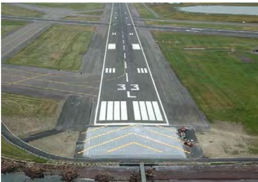
Figure S-2 Existing Runway 33L End
