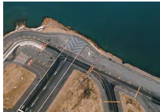
Figure S-3 Existing Runway 22R End
