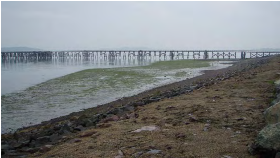
Figure S-6 Existing Eelgrass Beds and Light Pier at the Runway 33L End
