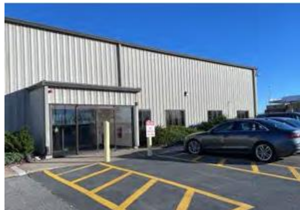
Entrance to Existing Maintenance Building
