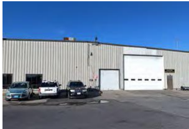
Side Doors to Existing Maintenance Building
