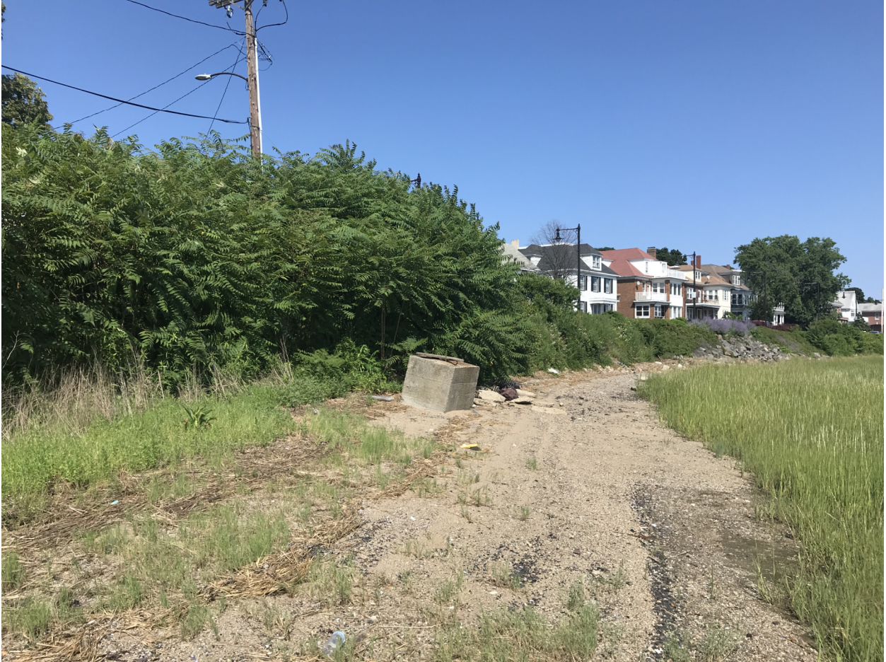
Figure 4: Existing Revetment along Bayswater Street facing Southeast
