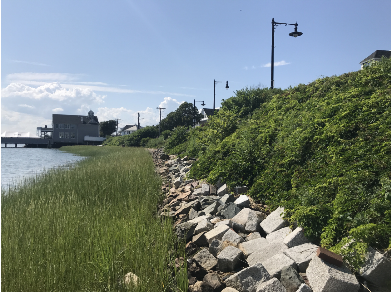
Figure 2: Existing Revetment along Bayswater Street facing Northwest
