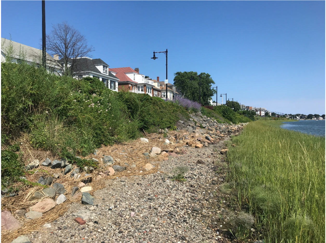
Figure 1: Existing Revetment along Bayswater Street facing Southeast
