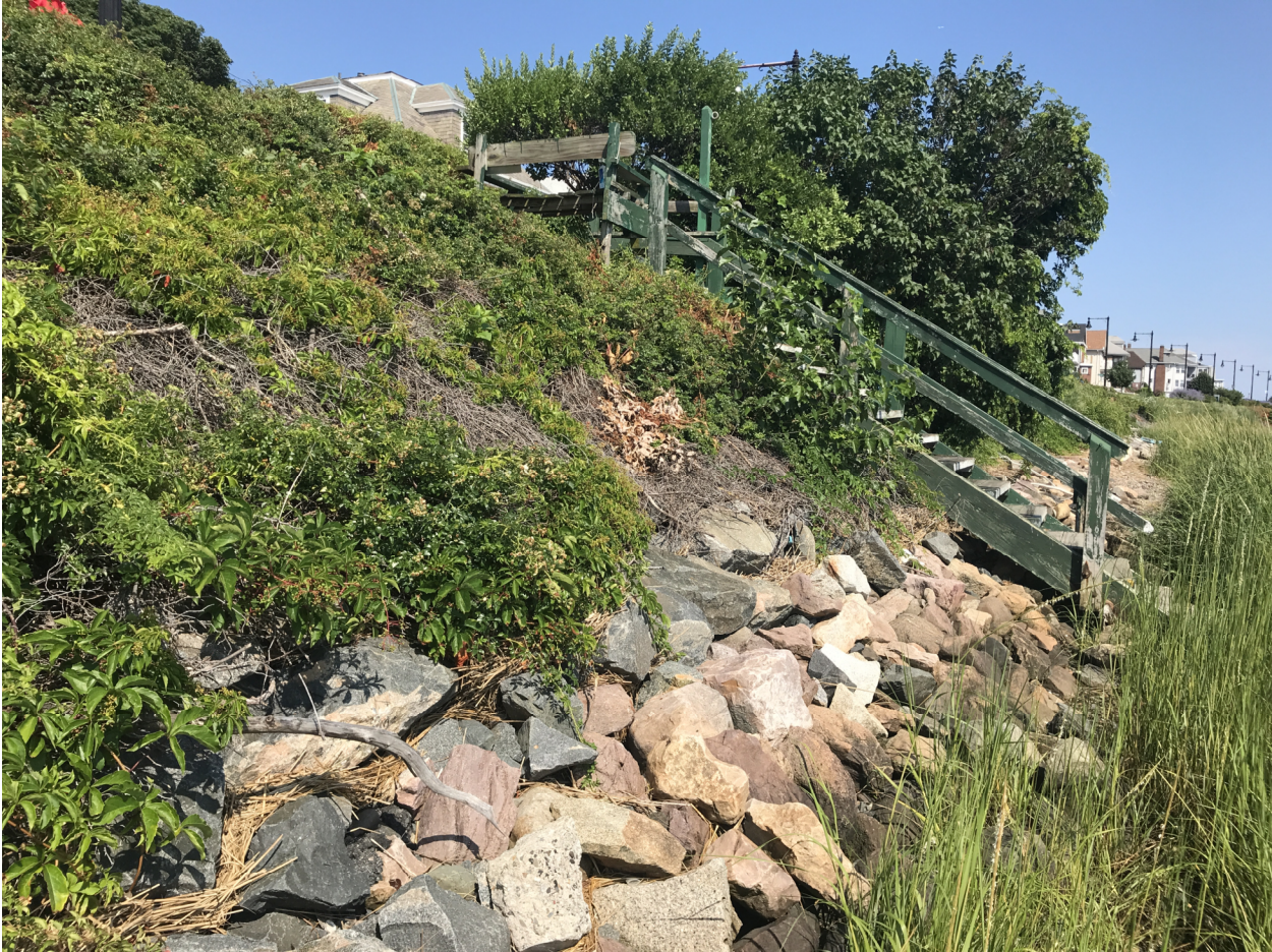
Figure 3: Existing Beach Access Stairway along Bayswater Street, facing Southeast
