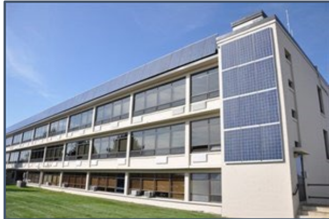
Figure 11-3. Solar PV Panels on Hanscom Field Terminal
