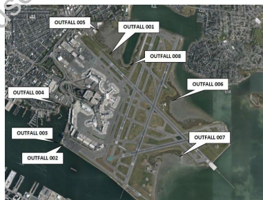
Logan Airport stormwater outfalls
