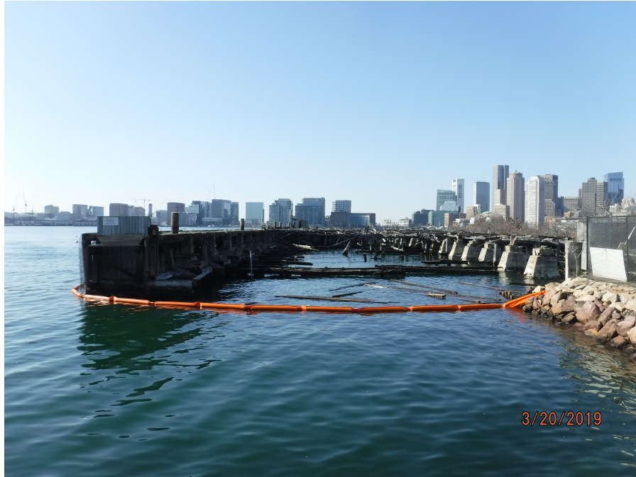
Photograph 1: View of the eastern side of Pier 3, facing south from Sailing Center.
