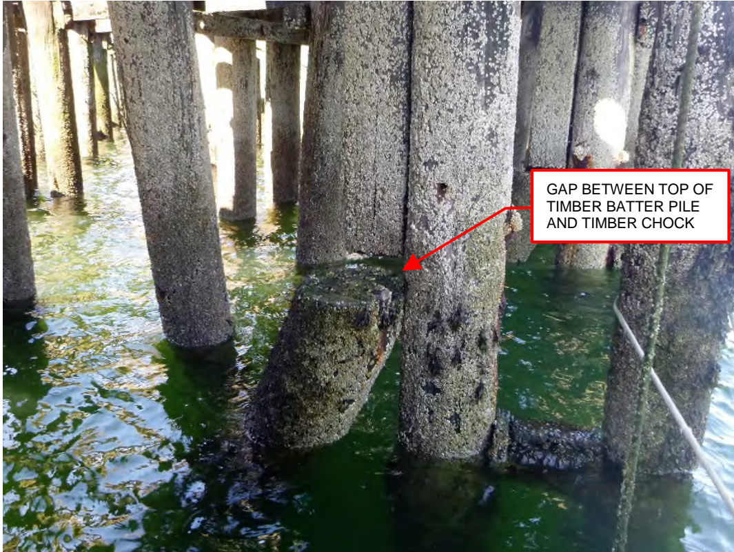
Photo 17 – Timber batter pile along southeast side of the pier.
