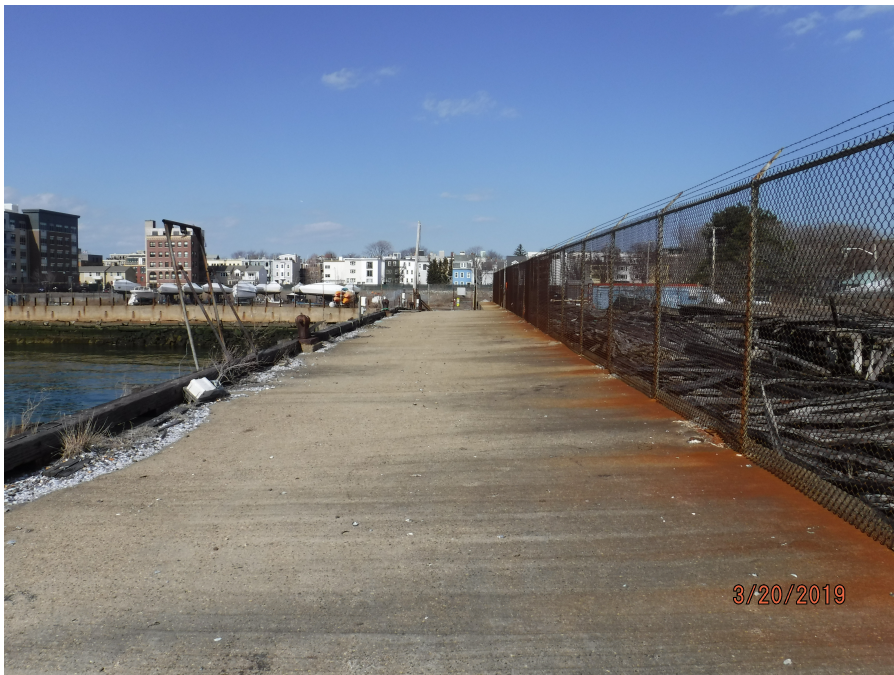
Photograph 6: View of the western apron along Pier 3, facing north.
