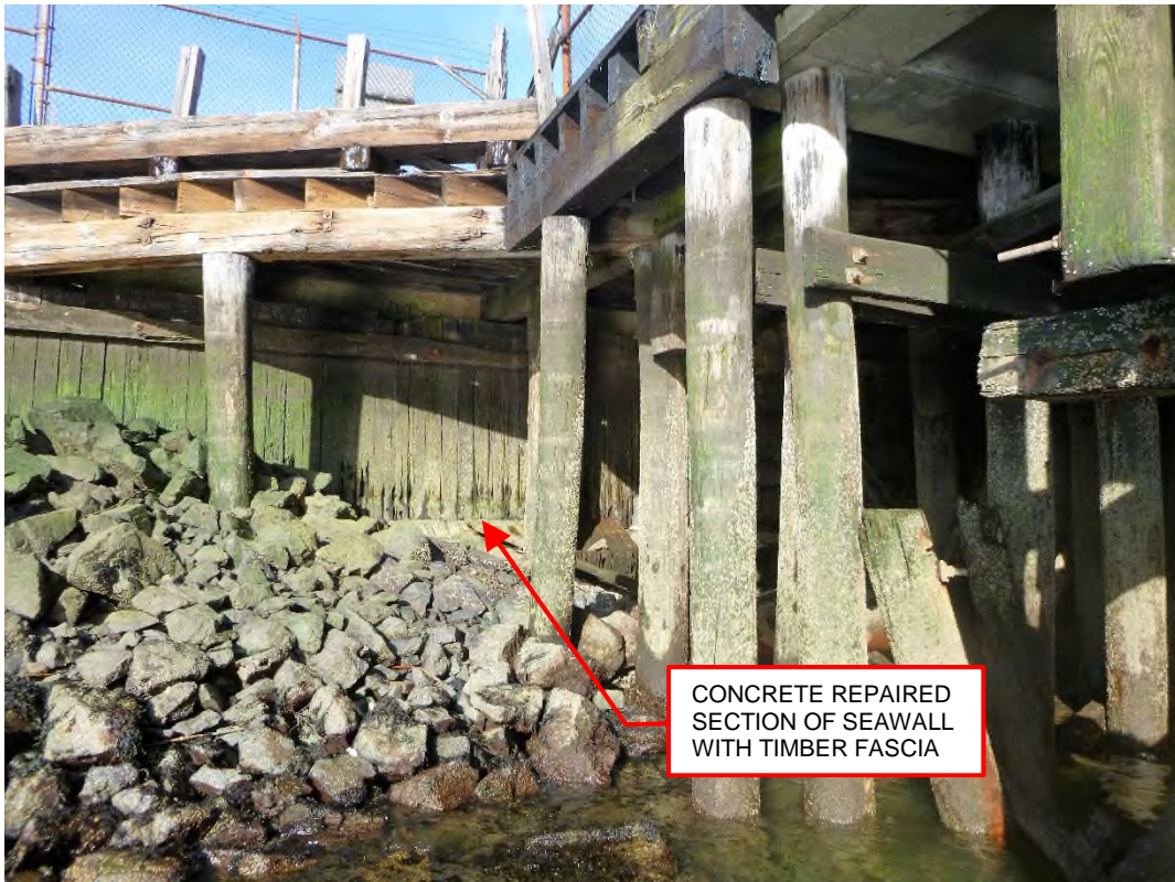
Photo 22 – Seawall with rip rap near the north corner of the pier.
