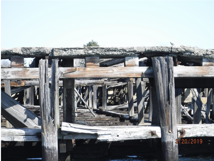
Photograph 7: Typical view of wooden and concrete piles/piers of Pier 3.
