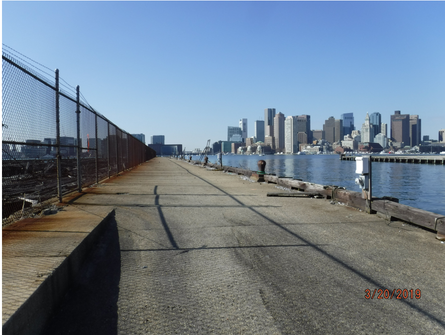
Photograph 5: View of the western apron along Pier 3, facing south.
