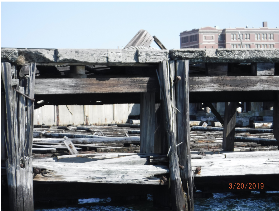
Photograph 8: Typical view of wooden and concrete piles/piers of Pier 3.
