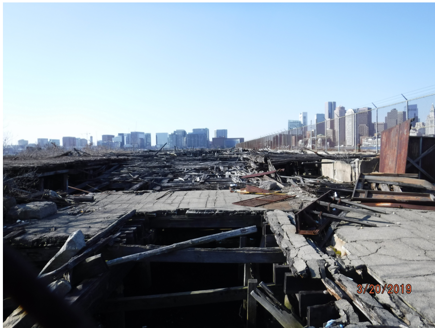
Photograph 2: View of the center of Pier 3, facing south from the backlands.
