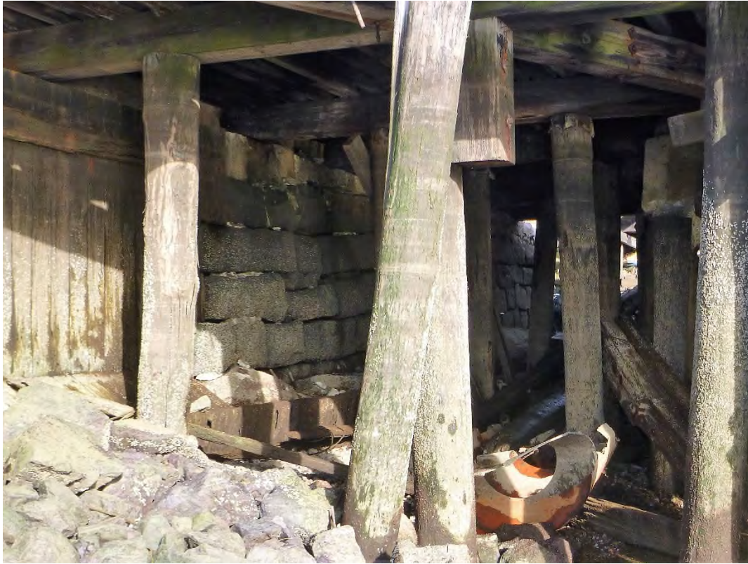
Photo 21 – Granite block seawall beneath pier near the north corner.
