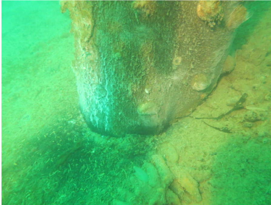
Photograph 11 : Typical view of subtidal piles/piers along Pier 3, and substrate bottom.
