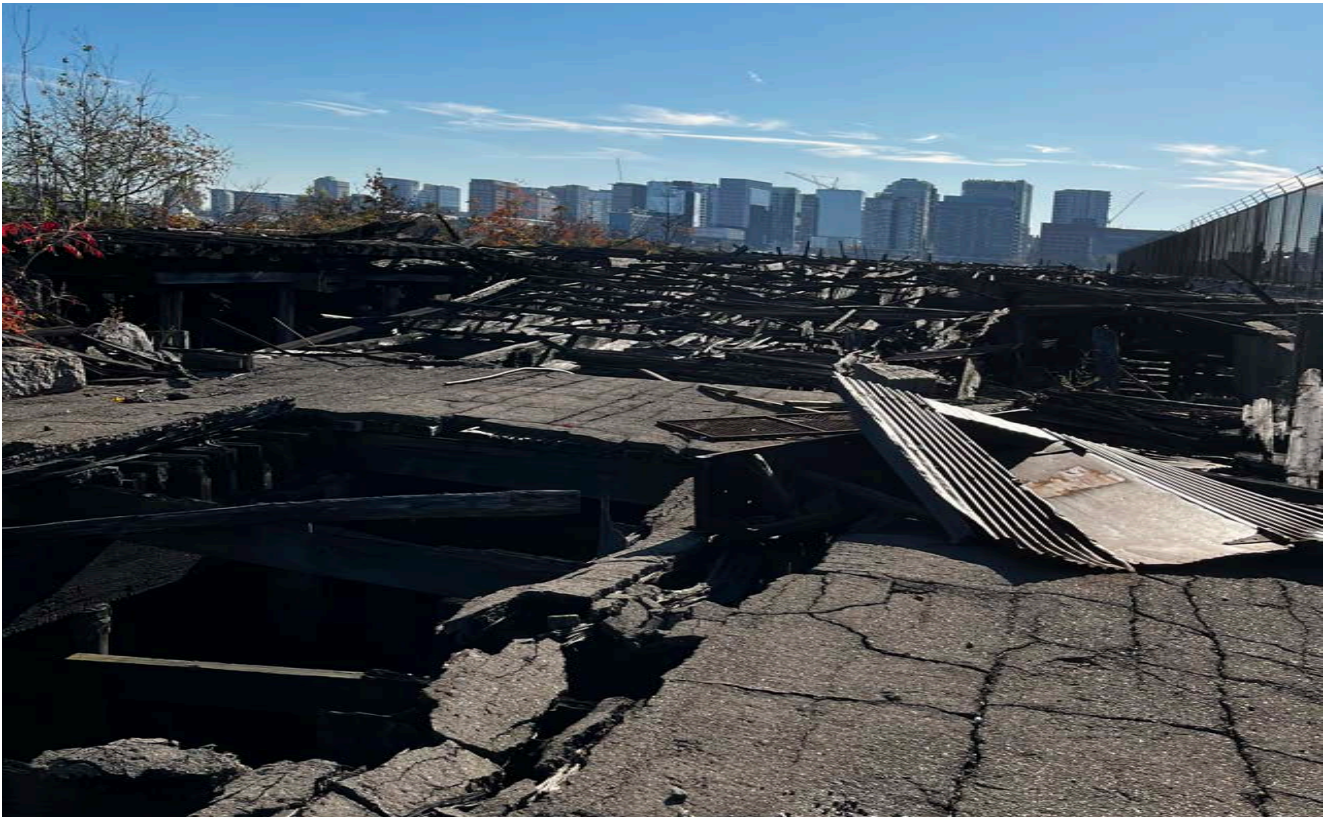
Photograph 5: Looking south from the concrete deck.
