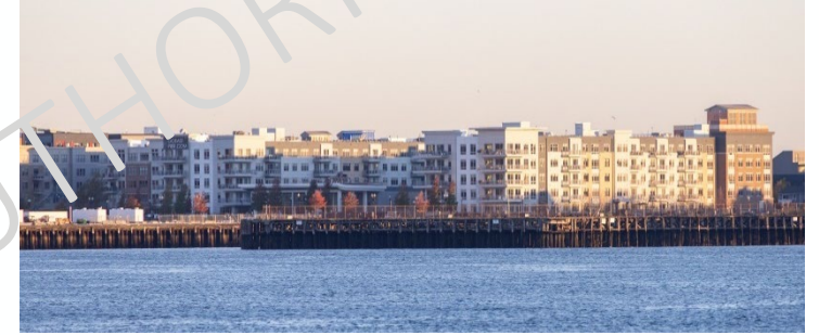
Portside at East Pier
