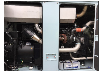
RTG crane engine
