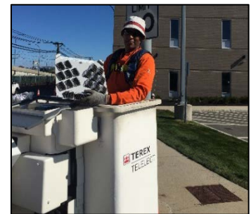
Retrofitting streetlights with LEDs
