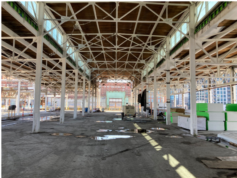
Commonwealth Pier Construction
