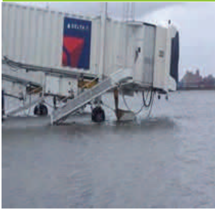
Hurricane Sandy: LaGuardia Airport flooded
