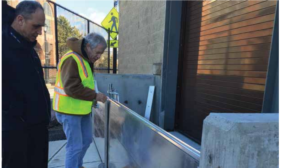
Flood barriers protect critical infrastructure at Boston Logan International Airport
