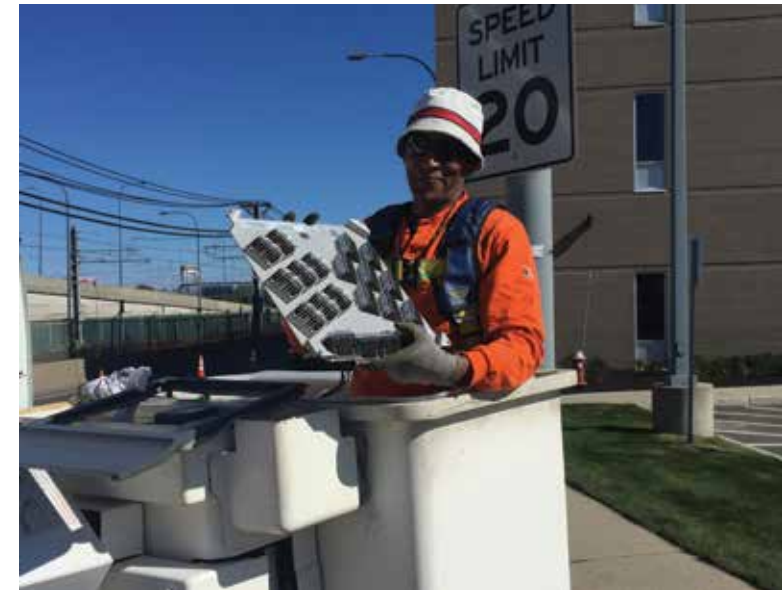
Installation of energy-efficient LED lighting at Boston Logan International Airport
