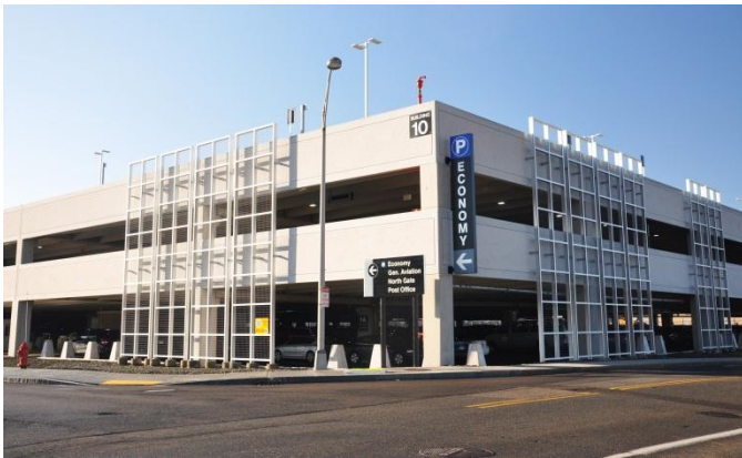
Economy Parking Garage. Source: Massport.
