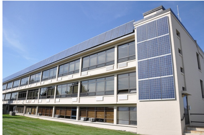
Solar Panels on Civil Air Terminal building. Source: Massport.
