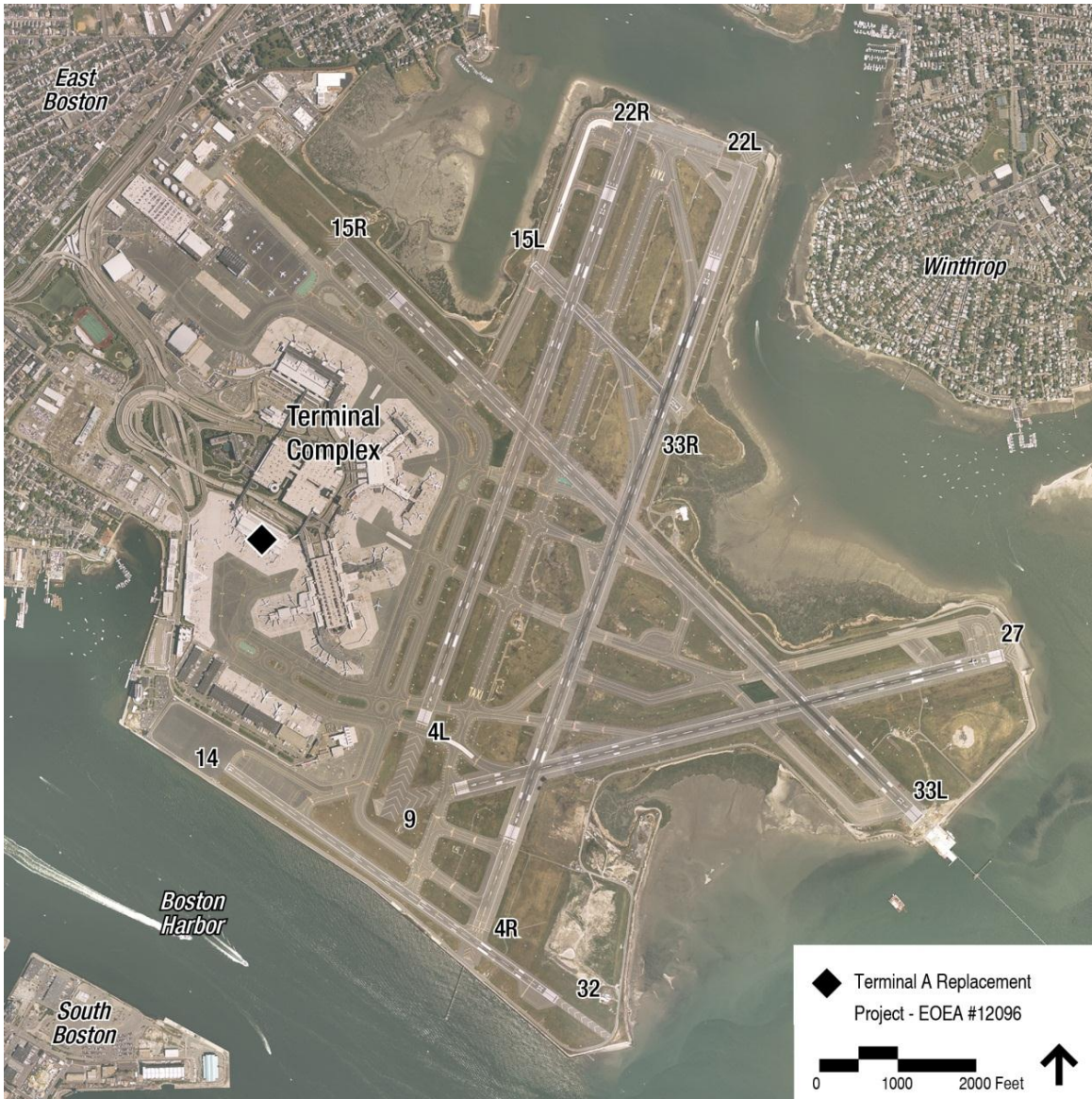
Figure 9-3 Replacement Terminal A Project
