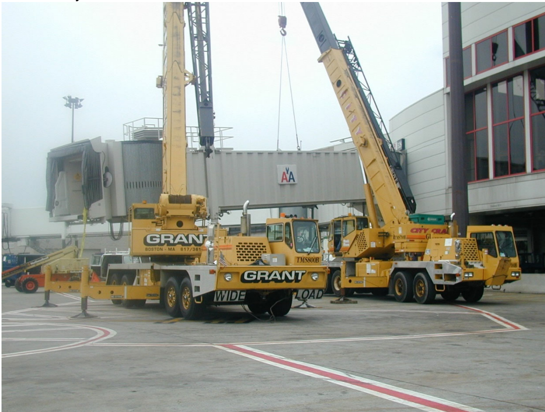
Jet bridge Work at Logan Airport
