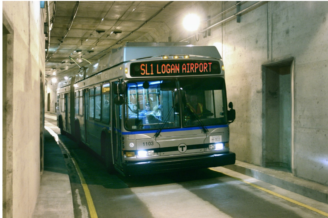
FIGURE 4: MBTA SILVER LINE POWERED BY TWO TROLLEY POLES DURING IN-TUNNEL OPERATION
