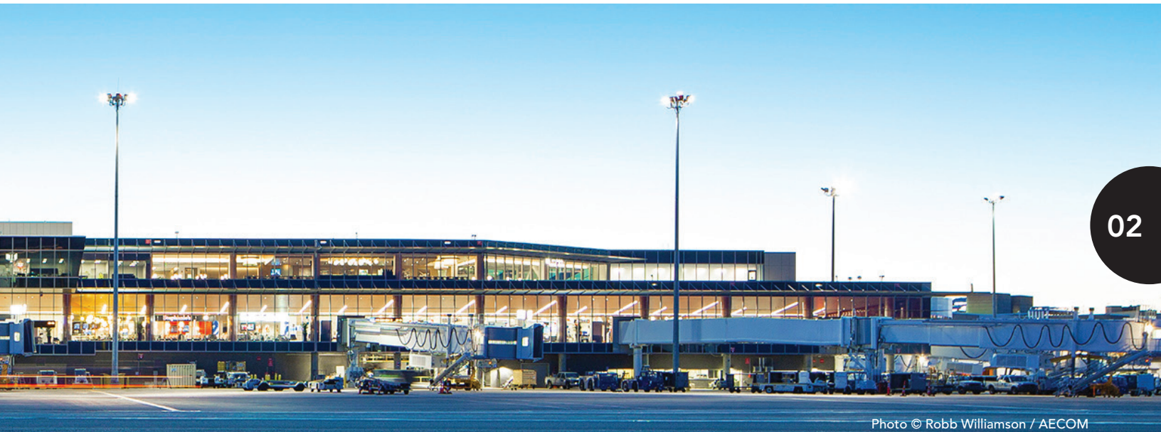
Photo © Robb Williamson / AECOM
