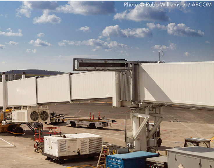
Photo © Robb Williamson / AECOM
